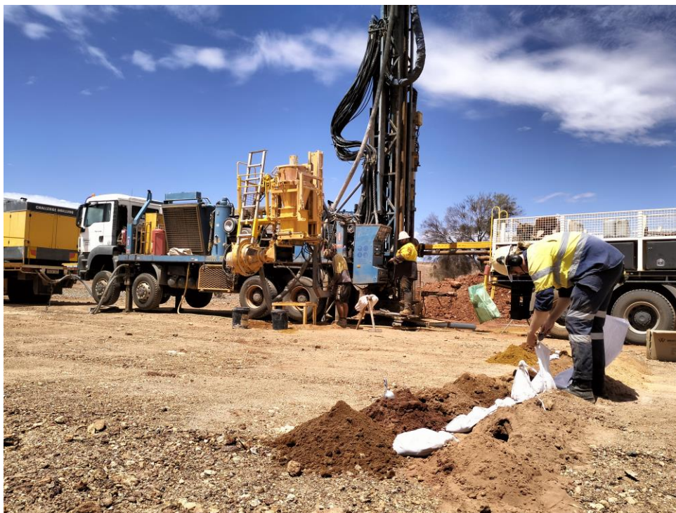
Figure (1): Reverse circulation drill rig on site at the Caledonian target.
